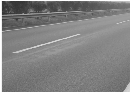
Fig. 4 Bleeding in overlapping area of SAMI
