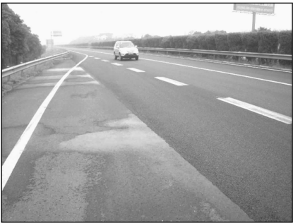
Fig. 6 Pavement permeability performance of AR-OGFC overlay after raining
