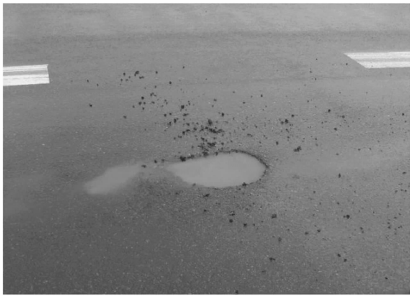
Fig.3 Overlay failure due to improper treatment of old pavement
