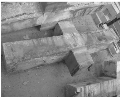
Fig. 3 Columns after rebar corrosion
