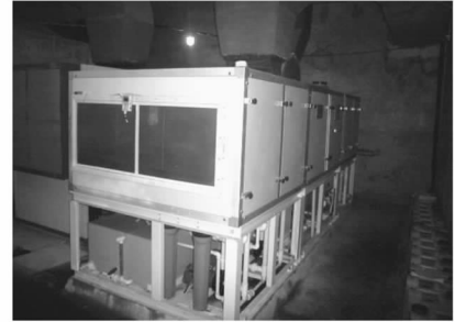
Fig. 3 Photo of liquid desiccant deep dehumidification processor
