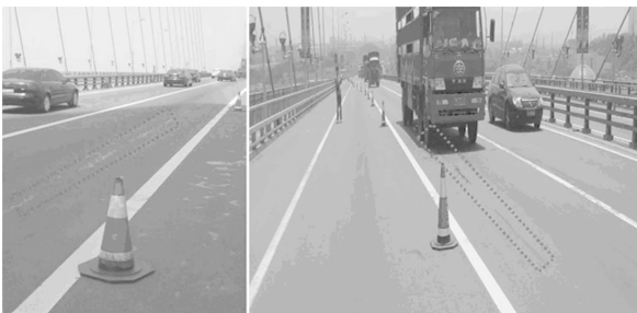
Fig. 2 Longitudinal regular cracks in the northbound drive lane on SNYRB
