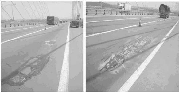
Fig. 7 Alligator crack in the southbound slow lane on SNYRB
