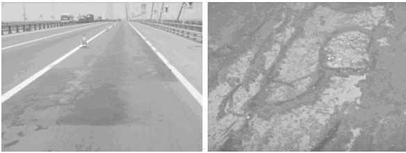
Fig. 6 Alligator crack in the northbound slow lane on SNYRB
