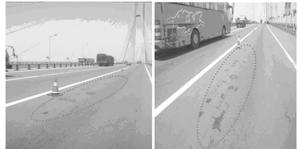
Fig. 4 Short hairline cracks in the northbound slow lane on SNYRB
