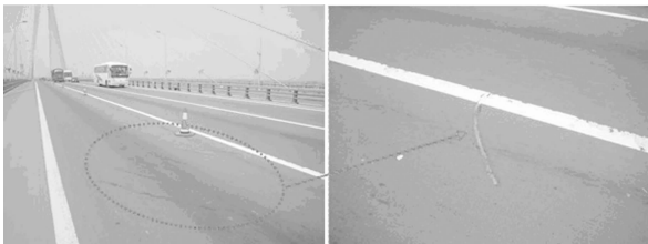
Fig. 10 Scratching on epoxy asphalt pavement on SNYRB
