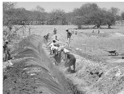
Fig. 7 Sub-surface dam construction, putting a PVC sheet (Irpaa)
