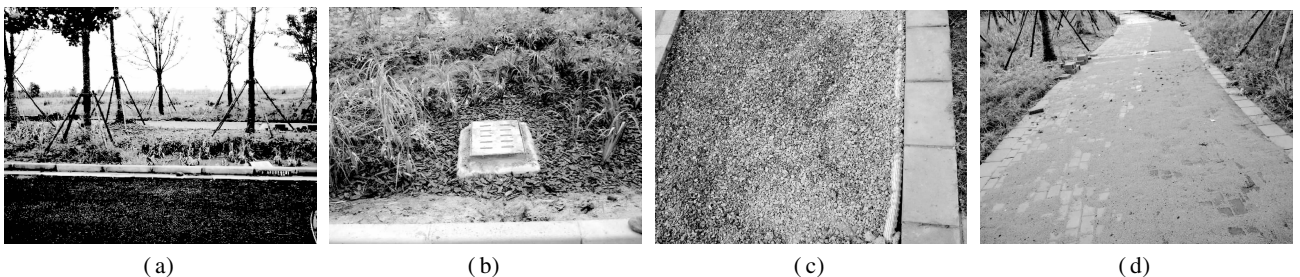
Fig. 6 Several LID practices implemented in this project. (a) Roadside bioretention; (b) Outlet of bioretention (overflow); (c) Permeable paving under construction; (d) Permeable paving before completion
