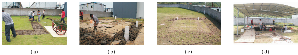
Fig. 2 Dewatering measurement during excavation. (a) Excavating a trench around the planned test square; (b) Setting two pumping wells at the two corners; (c) Backfilling the trench with sand and gravel; (d) Building a protective shed above the planned test square
