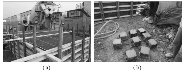
Fig. 5 The site of concrete casting. (a) Low-strength concrete; (b) Concrete cubes
