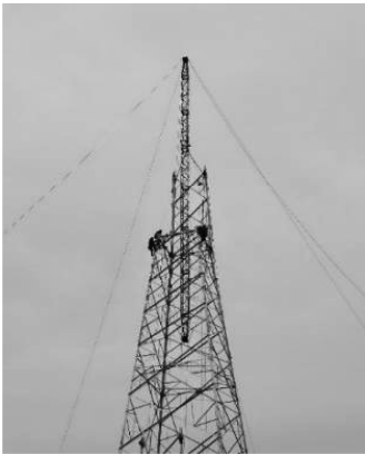
Fig. 3 Construction site of the suspended derrick
